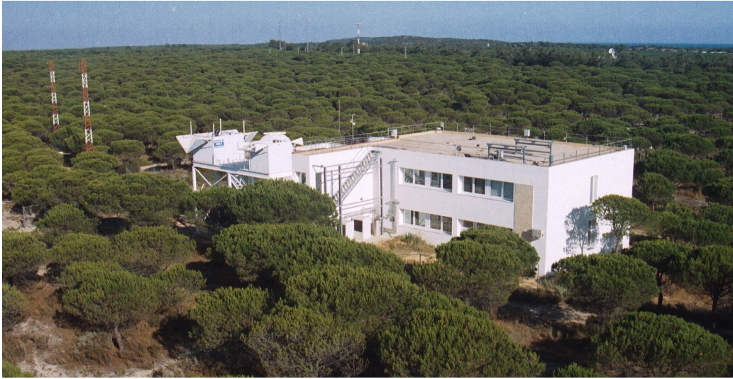
Figure 30 The building of ESAt with domes of BOOTES-1A and BOOTES-1B (2002).
